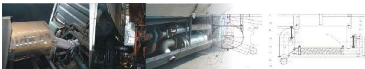
50. Figure: Flue gas treatment systems with an exhaust resistance of up to 2-9 mBar OEM conventional systems can result in fuel savings of up to 15-25% compared to 250-450 mBar counter-pressure [4]
