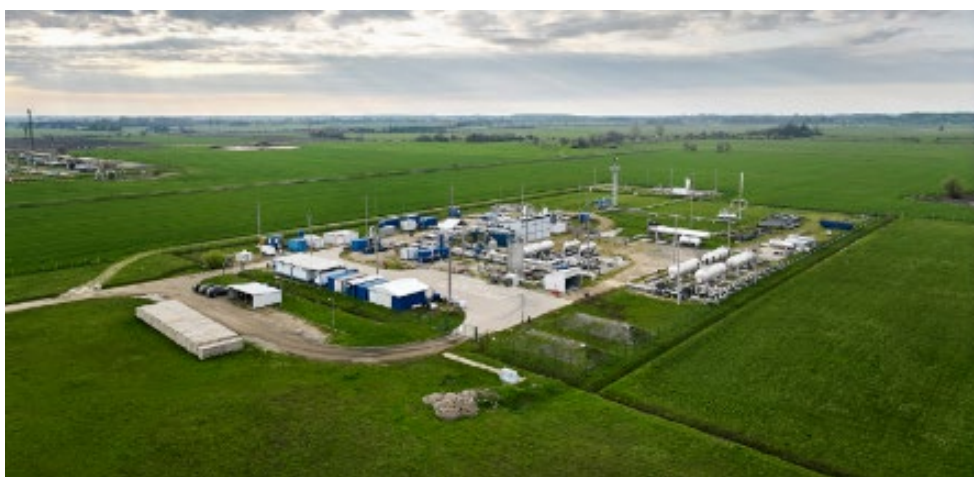
23. Figure: The gas extraction site in Endrőd [18]
