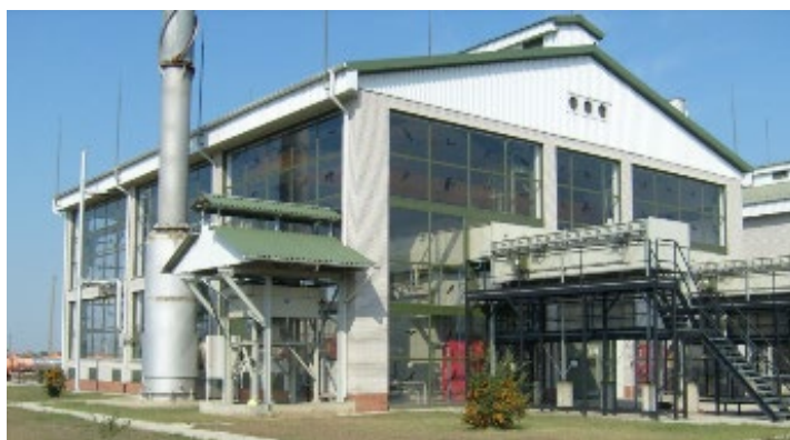
35. Figure: Natural gas pressure boosting site, Szolnok [3]
