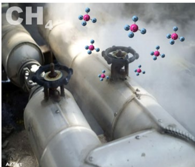
11. Figure: All pipe connections and fittings can be a source of methane leakage. [4]
